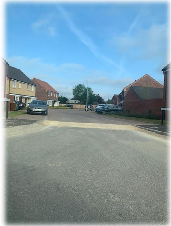
Figure 10: View towards a cul-de-sac
