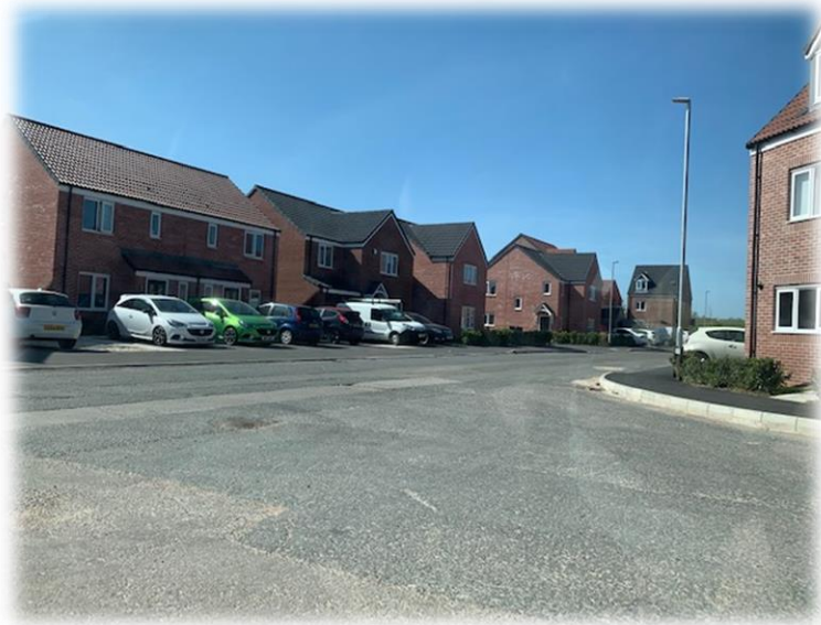
Figure 7: View of front of plot parking which over dominates the street scene in this particular location
